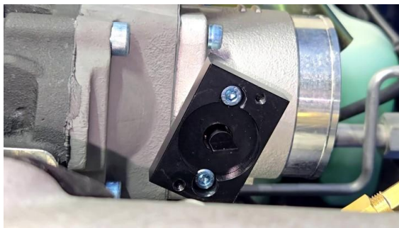
A - Extension installed
